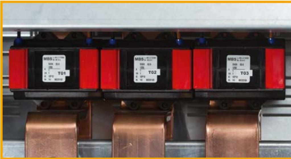
**Fig. 9** Protection current transformer set
