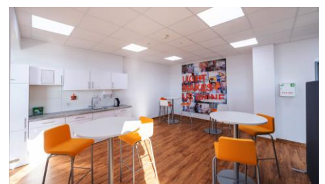
Community room with ZIGBEE light and sensor control
